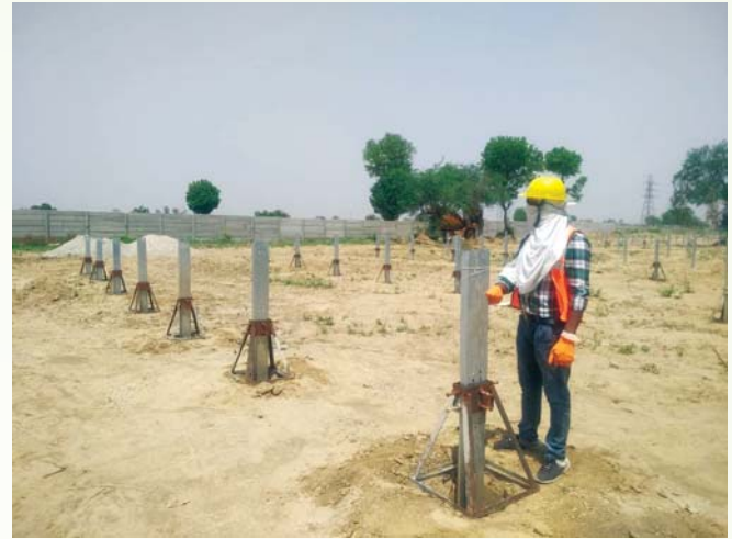
Piling and Foundation work at 2 MW solar site at Diwana
